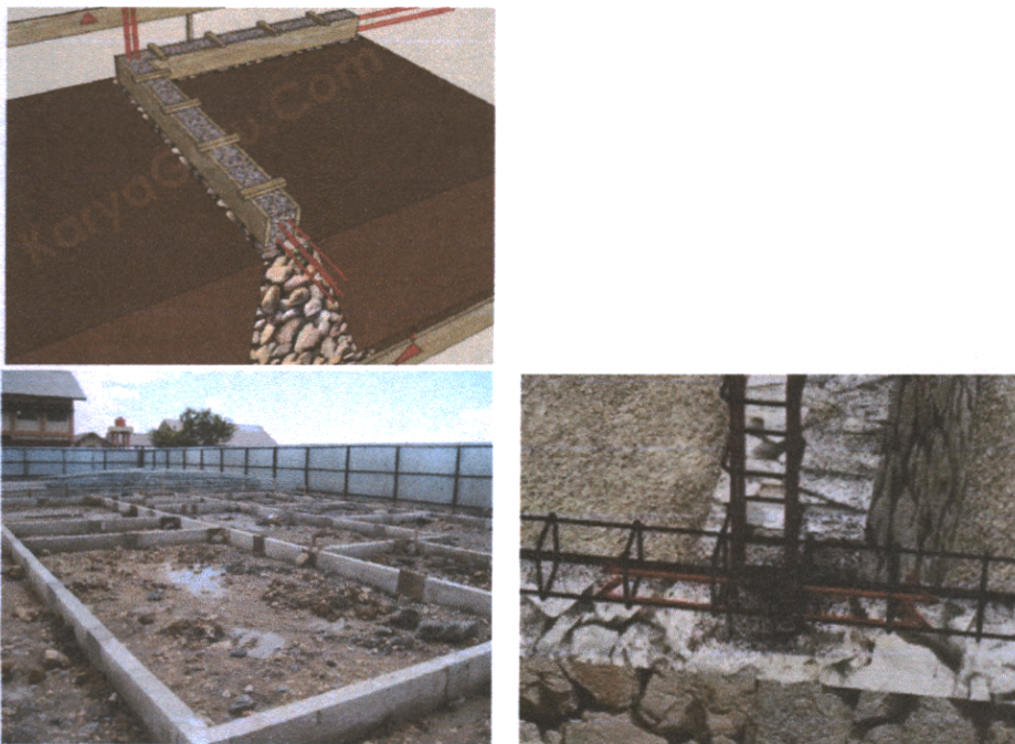
Gambar 2.24; Sloof Beton
